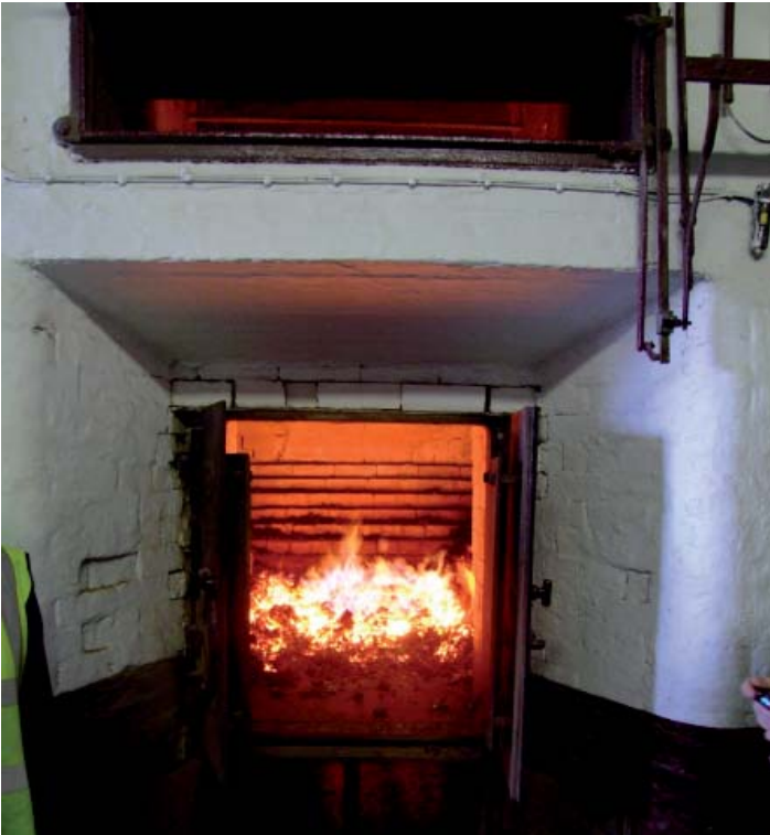
Kiln / The Balvenie. Photo Credit: Neil Wilkie
